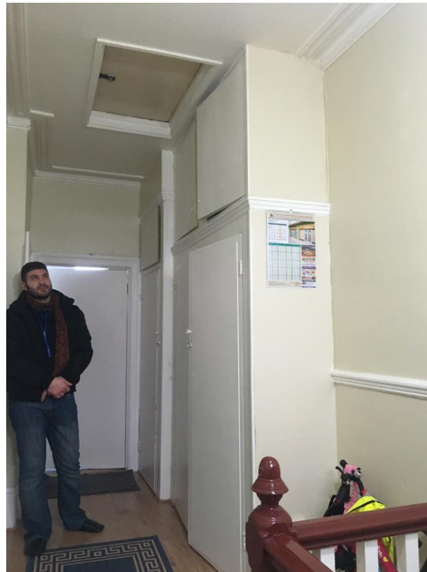
Wardrobes to First Floor Landing
