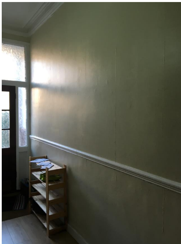
Communal Entrance Hall in fair condition with no obvious cracks
