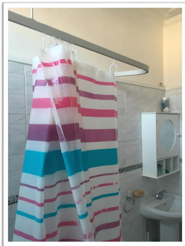
Bathroom wall on First Floor appears in fair condition
