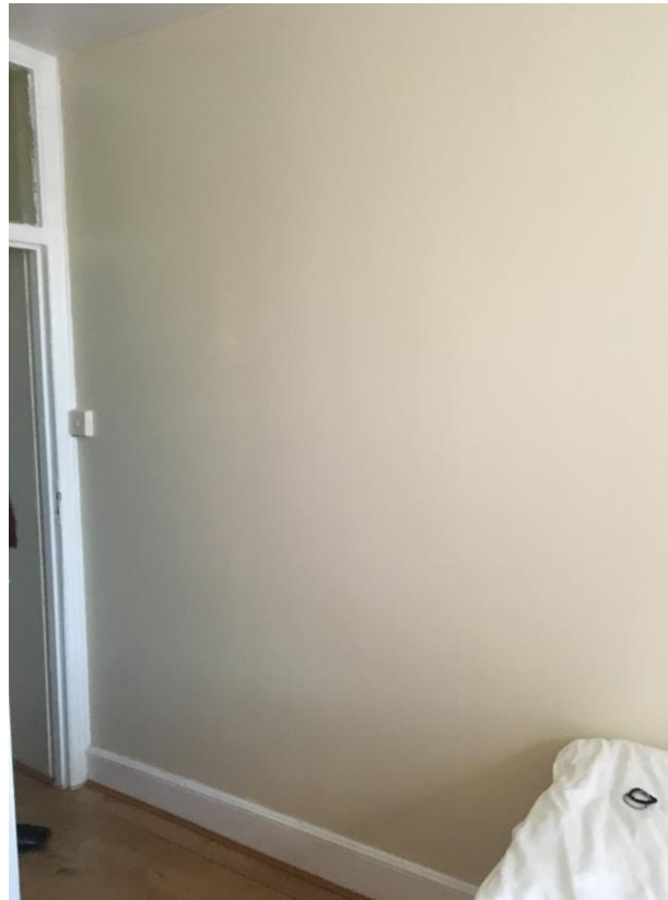
Wall to rear bedroom appears in fair condition
