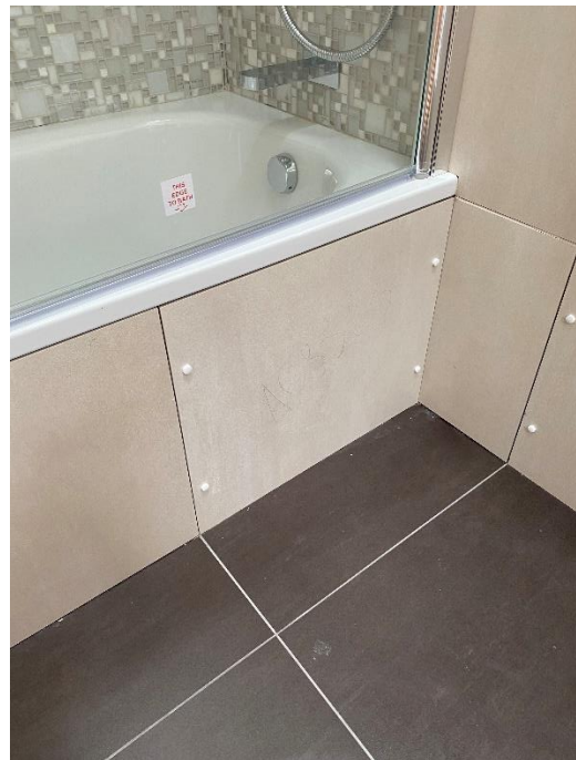
New Bathroom pending completion
