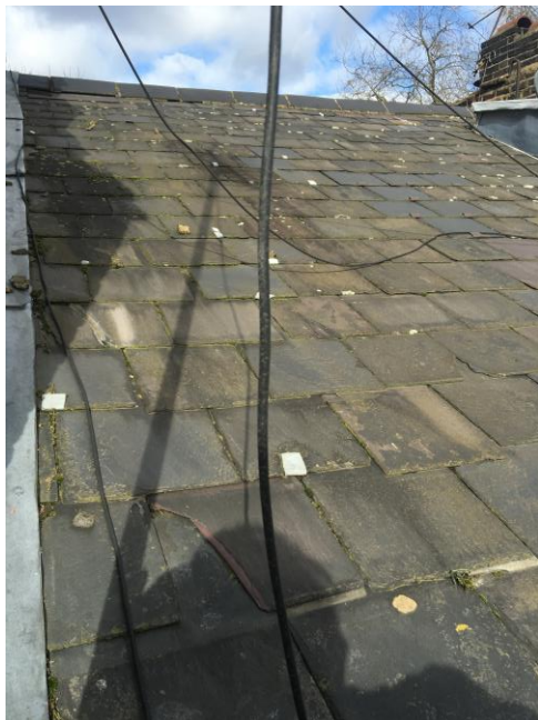
Damaged Slates Prior to re-roofing works Regular supervision provided good levels of workmanship
