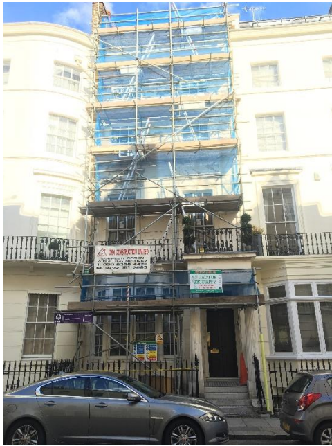
Stanhope Place Fully Scaffolded
