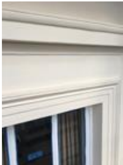
Detailed regular supervision following repair
