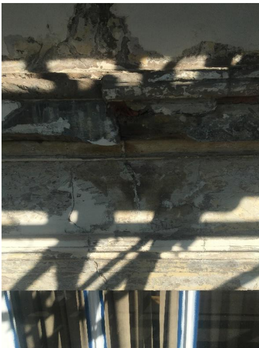
Decorative Stone Lintel detail
