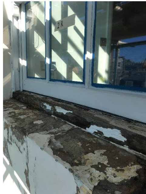
Windows completely stripped back for effective repairs
