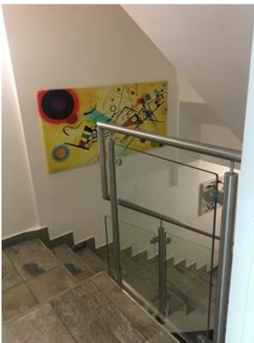
Access to the offices below at basement level
